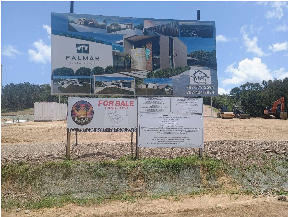
Sign located at the Site entrance main gate depicting NPDES ID Number PRR1000JG.
