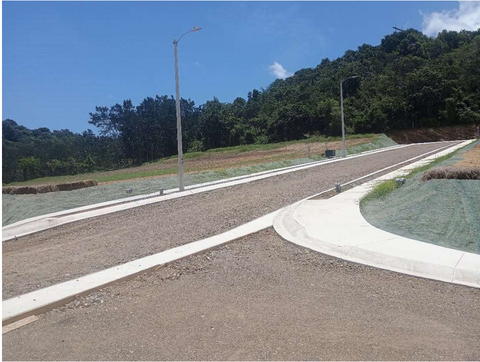
Main access road with temporary stabilization with gravel to prevent further erosion. View of the slopes with erosion control blankets and hay bales installed.
