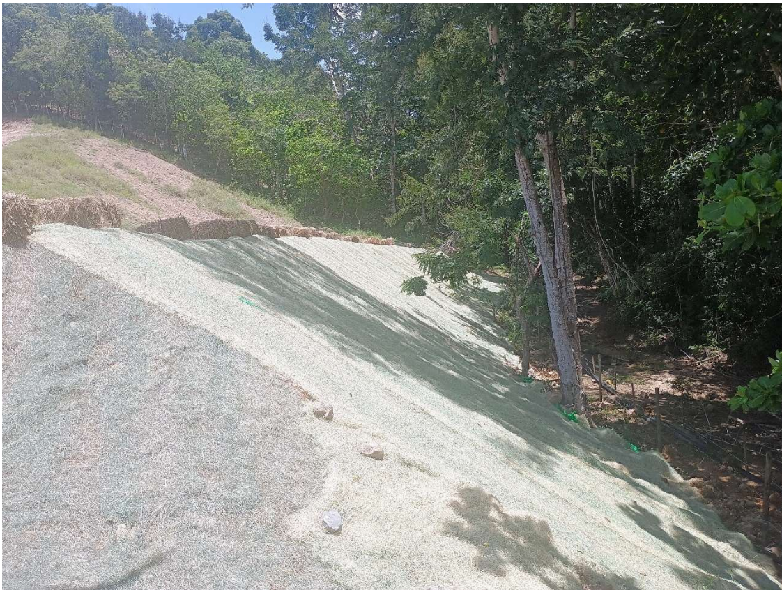
Another picture of the southeast part slope with erosion control blanket installed
